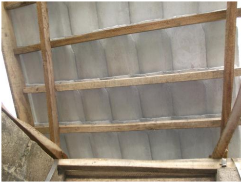
Fig 10: Interior of the roofing
