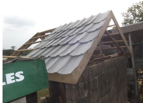
Fig 9: Installation of roofing tiles
