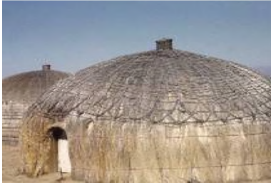
Figure 3. Zulu beehive house built of rope lattice, thatch and wooden strips.
