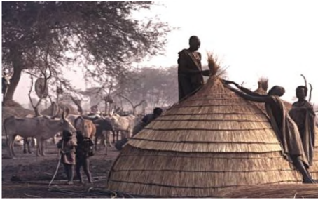
Figure 4. Eastern African nomadic shelter of stick framework covered with hatch.
