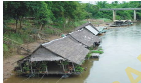
Figure 11. Local building at riverine area built with wild coconut timber framework and raffia palm leave roof covering.
