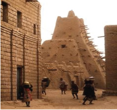
Figure 1. Indigenous building of Songhai in Mali.
