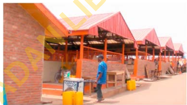
Fig. 10. Transformation of the Old Market to New One. One of the Prototype Neighbourhood Markets in Akure Built Between Nov 2010 and April 2011 by the Current Administration in Ondo State, shown as M3 on Fig. 8b and Table 4. (Source: Researcher).
