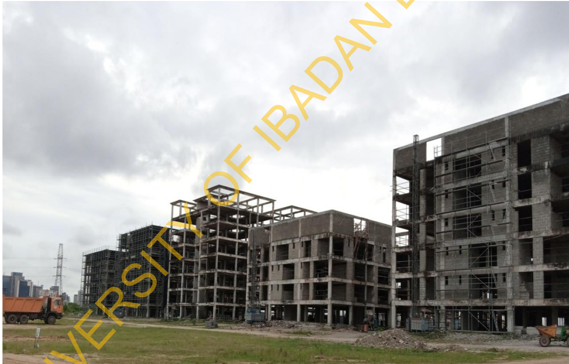
Fig. 4.9: On-going Construction of the new Commercial, Residential and Leisure Community
