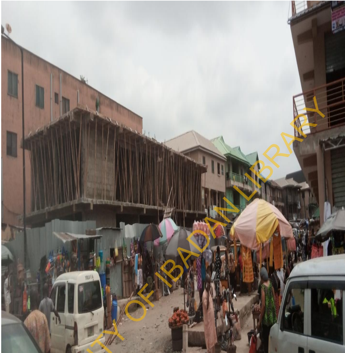
Fig. 4.25: An On-going Construction of a Shopping Complex in Oshodi
