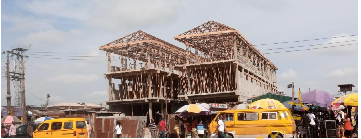
Fig. 4.29: An on-going shopping complex in Alimosho LGA
