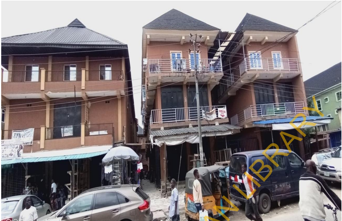
Fig. 4.24: Some Newly Constructed Shopping Complexes in Central Oshodi
