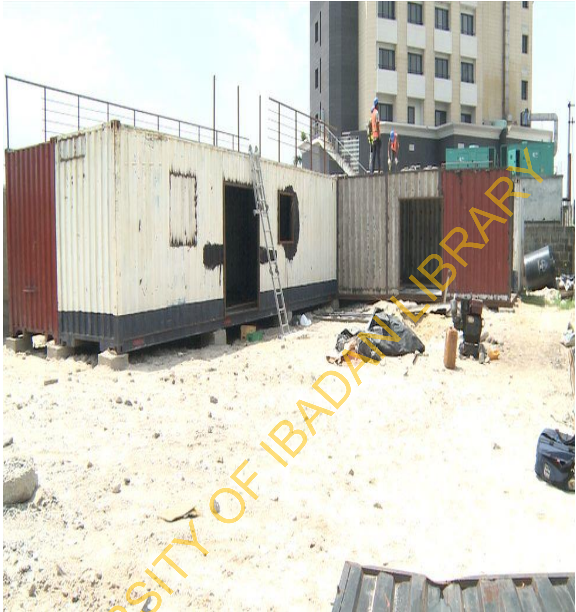
Fig.4.41: Construction of containers for commercial purposes
