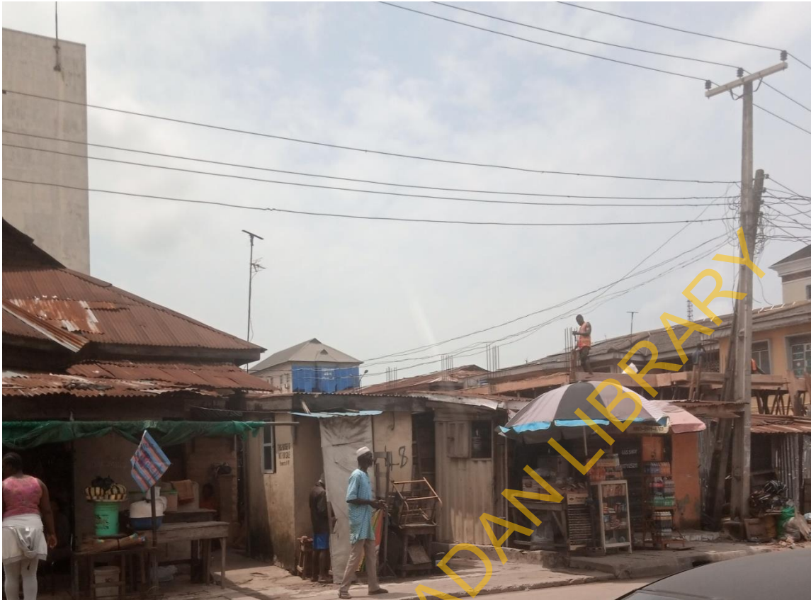
Fig.4.33: Image of an on-going high rise building in Yaba
